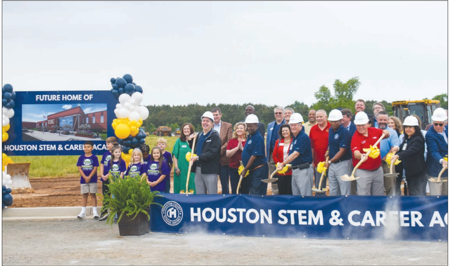
Community leaders gather Friday, May 1 for the groundbreaking ceremony. The expected completion date is August 2027.
